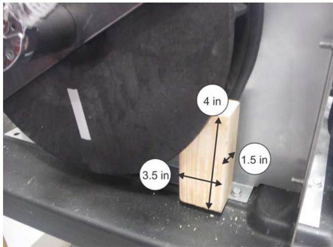
FIGURE 66. BLOCKING THE ALTERNATOR FOR INSTALLATION
